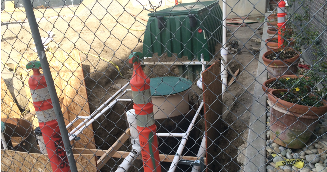
Graywater tank being installed outside of the LACI LaKretz Innovation Campus
