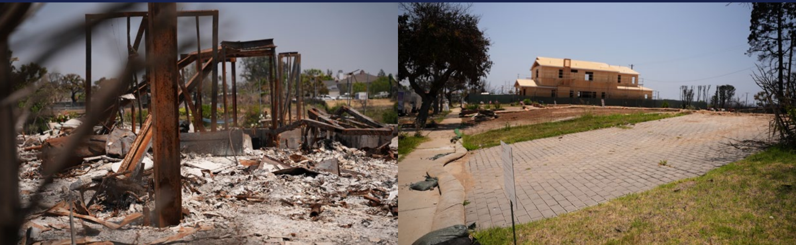
Home burnt down in the Pacific Palisades Fire (left). New home construction in the Pacific Palisades (right).
